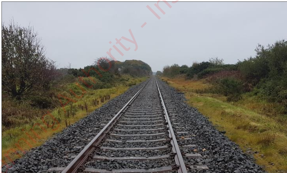
Figure 18. Survey Point 7 – View to Southeast
