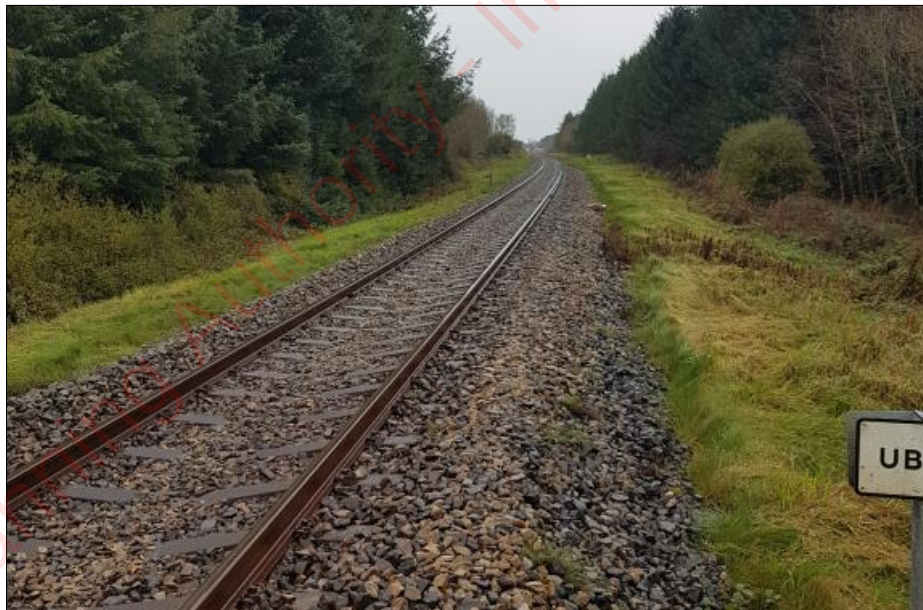
Figure 6. Survey Point 1 – View to Southeast
