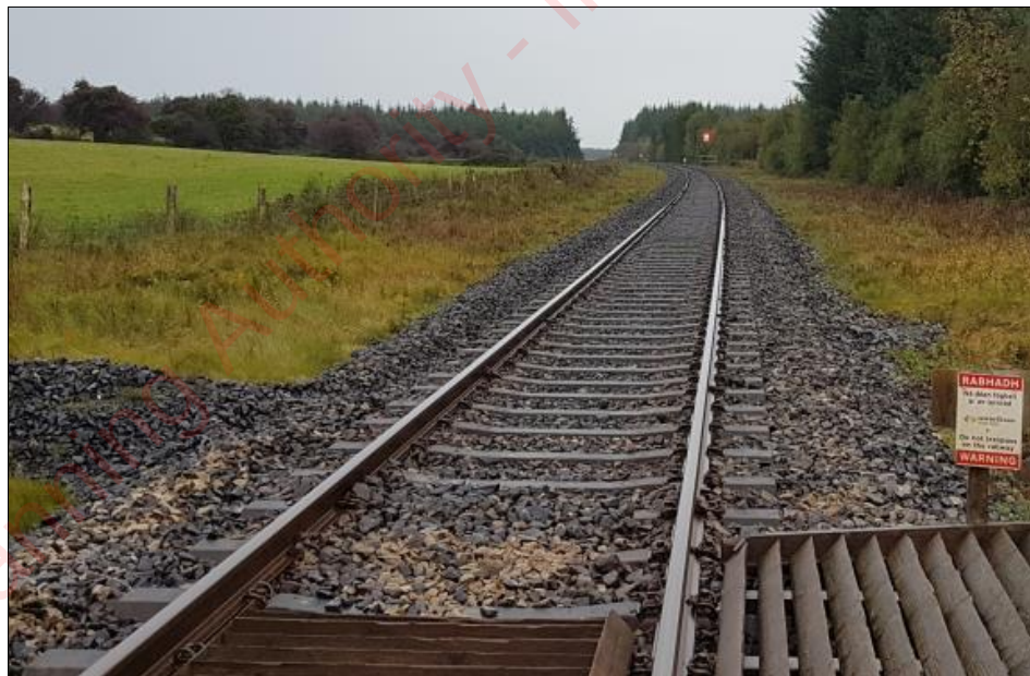
Figure 10. Survey Point 3 – View to Southeast
