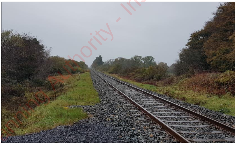
Figure 16. Survey Point 6 – View to Southeast
