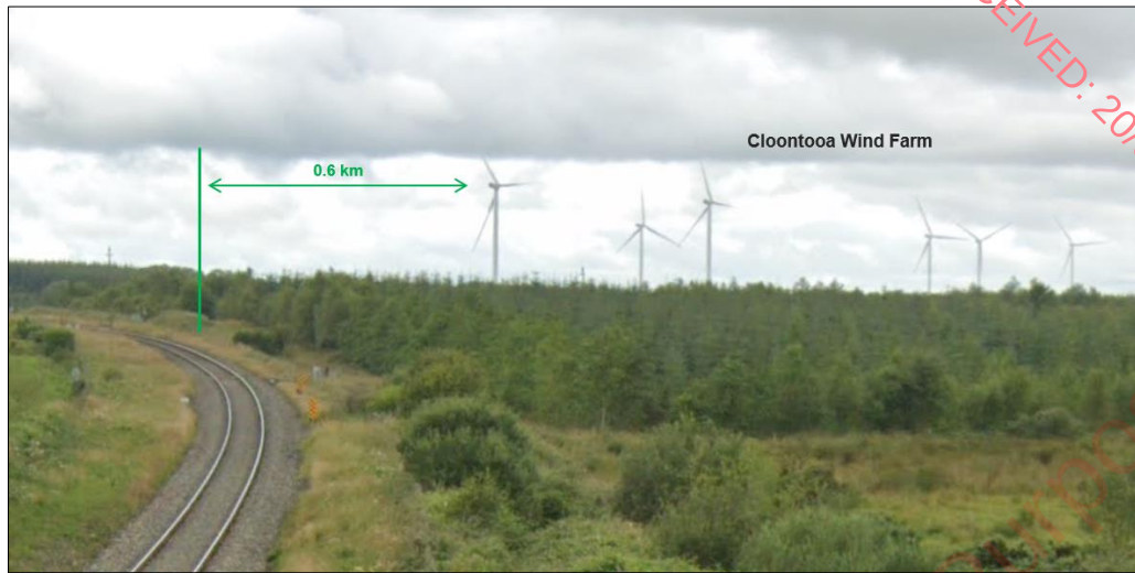
Figure 22. Cloontooa wind turbines shown relative to Irish Rail track
