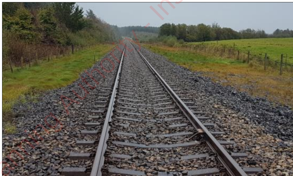
Figure 8. Survey Point 2 – View to Southeast
