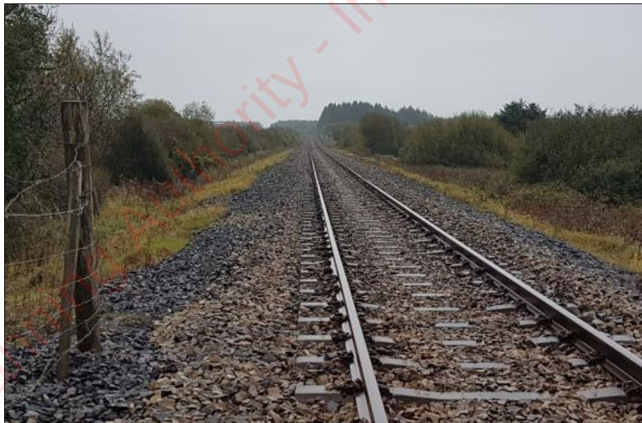
Figure 12. Survey Point 4 – View to Southeast
